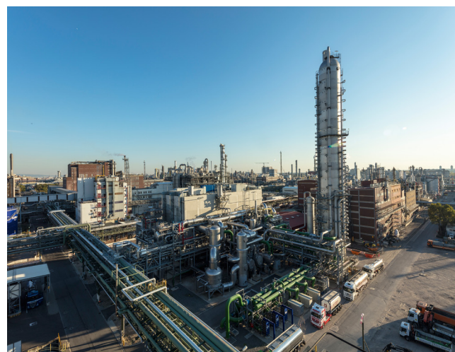
Demand for platinum in the production of nitric acid is expected to recover strongly in 2023. Picture credit: Nitric acid plant, BASF
